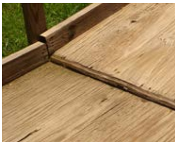
Uneven, bumpy transitions, warped slick surface.
